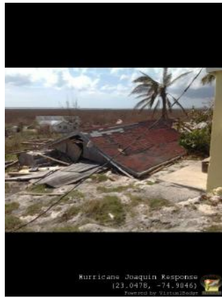
Completely Destroyed Home 23.0478, -74.9046
