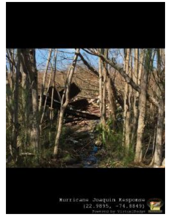
Completely Destroyed Home 22.9895, -74.8849
