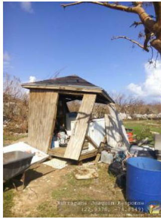
Partially Destroyed Home 22.9378, -74.8849
