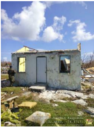
Partially Destroyed Home 22.8863, -74.8717
