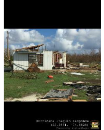
Completely Destroyed Home 22.9831, -74.8828
