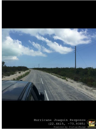
Power Poles All OK
