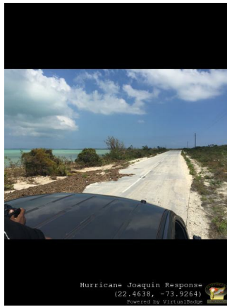
Debris on Road
