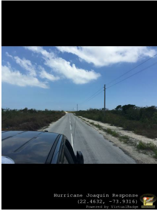
Power Poles All OK
