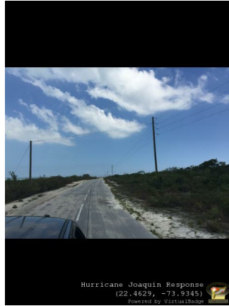
Power Poles All OK
